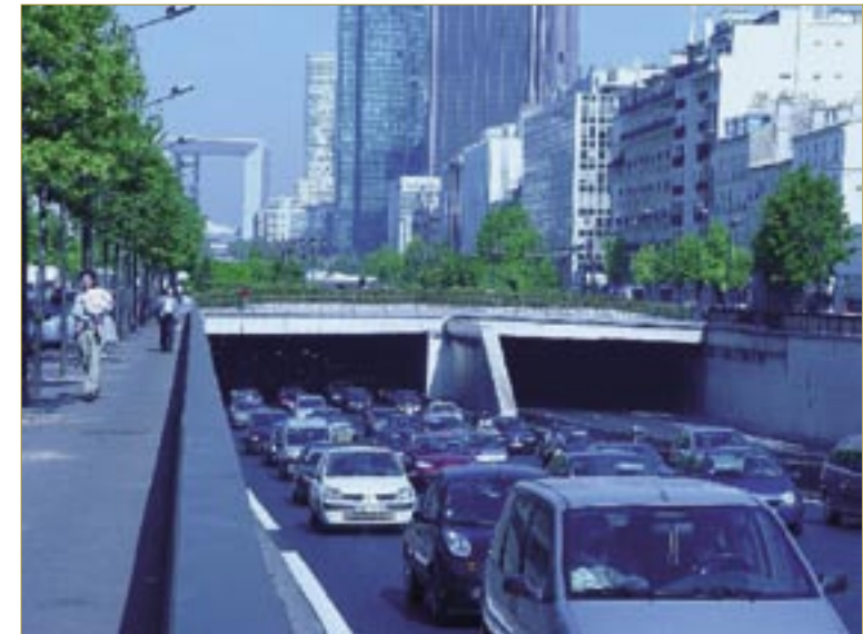
Example of traffic density in an urban tunnel
